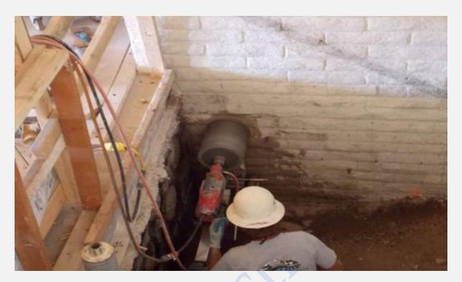
Core Drilling for Heating and Cooling Pipe Pathway
